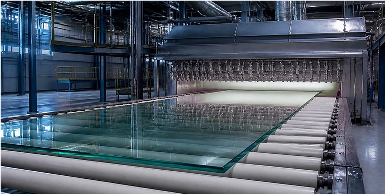
TEMPERING LINE — QUENCH SECTION
