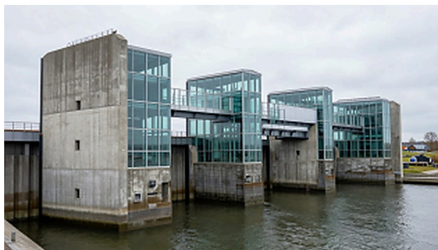
Storm Surge Barrier
