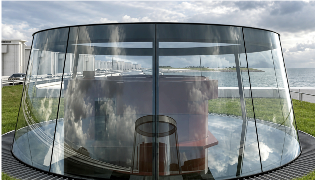
Den Oever Pumping Station
